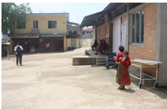
Gorkha District hospital. Building closest right hand side is the Emergency room with the dental ward attached. White building is the OPD building with pharmacy and X ray underneath.
